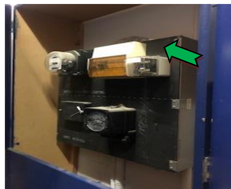
16. Just Sports, interior, ground floor, eastern elevation, switchboard – non-asbestos containing bituminous backing board.
