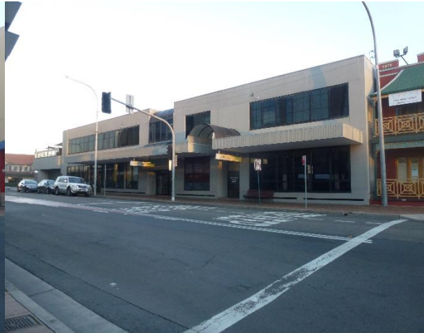
Figure 16: Two storey commercial building at the intersection of Scott and Terminus Street
