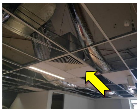
6. Council Offices, interior, ceiling space, throughout – synthetic mineral fibre containing compressed ceiling tiles.
