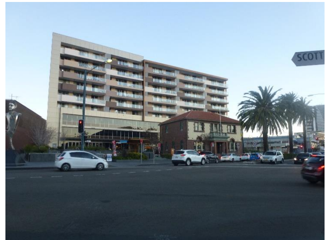
Figure 20: Nine storey mixed use residential building to the west
