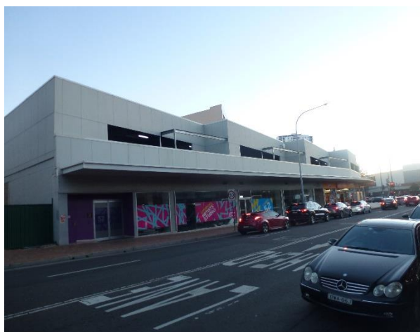
Figure 4: Commercial building occupying the site as viewed from Scott Street (north east)
