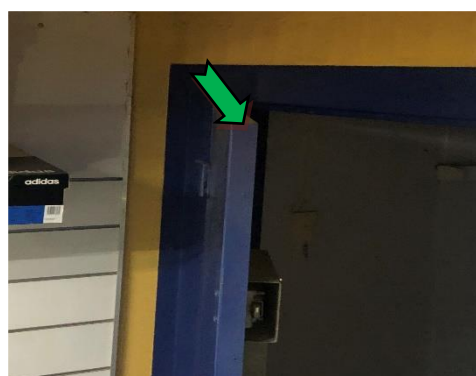
17. Just Sports, interior, ground floor, north-eastern elevation, safe door – assumed non-asbestos containing internal insulation.
