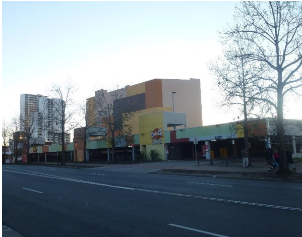
Figure 6: Above ground car parking structure as viewed from Terminus Street (south east)
