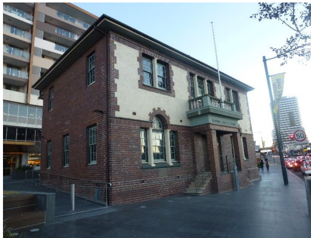
Figure 19: Memorial Arts Building
