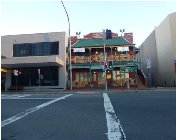
Figure 15: Two storey commercial building to the east of the George Street through site link
