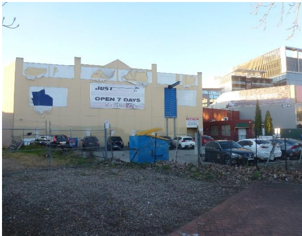
Figure 8: Rear car park of the commercial building as viewed from Terminus Street (south east)
