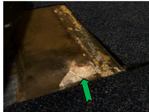
14. Just Sports, interior, under carpet, floor – non-asbestos containing screed.
