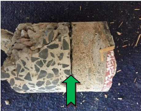
9. Surgery, interior, throughout, floor core sample – non-asbestos containing bituminous material.
