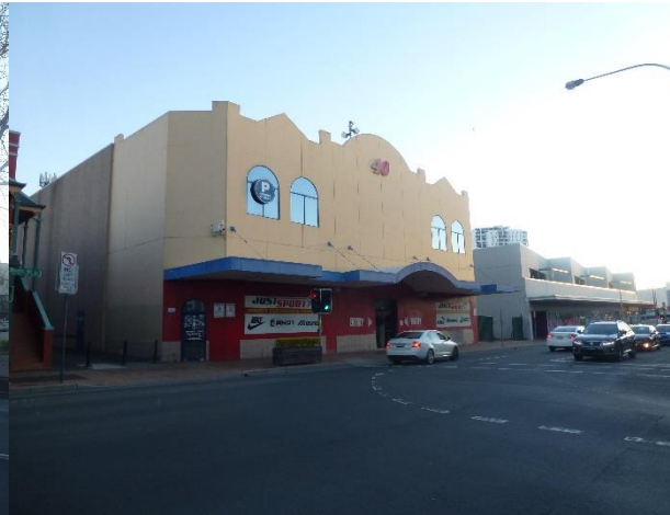
Figure 7: Commercial building occupying the site as viewed from Scott Street (north east)
