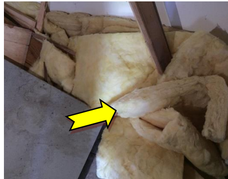
10. Surgery, interior, back room adjacent kitchenette, insulation batts- suspected synthetic mineral fibre insulation.
